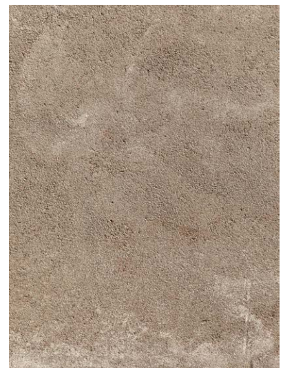
Detail of a wall, Christiansborg Slotskirke
