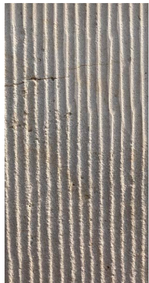
Detail of a wall, Vindebrogade
